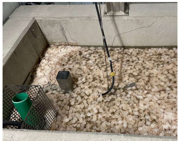
Mutag BioChip 30™ in the biofilter of the RAS system (denitrification stage)
